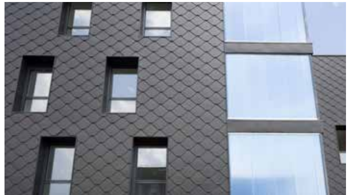
Architect: Rocheteau & Saillard
